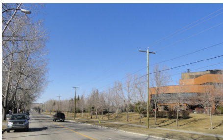
Figure 1. Hanging power cables in a road corridor in Canada
