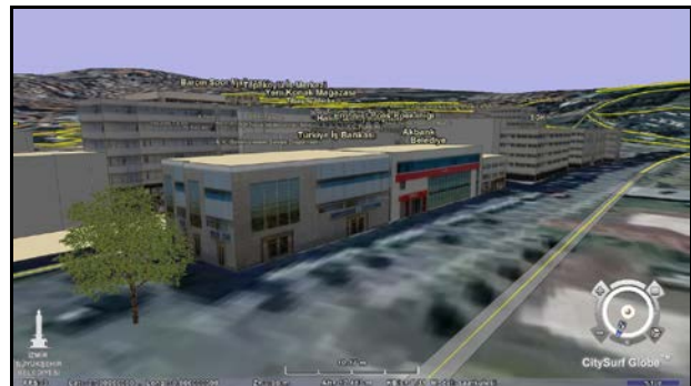
Figure 10. Surroundings of banks Source: CitySurf, 2011
