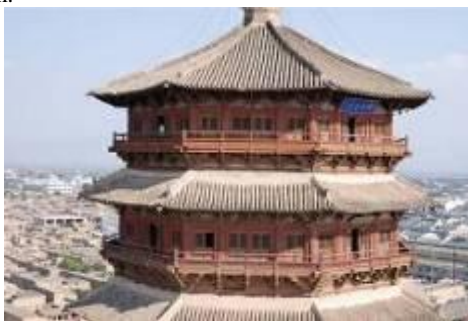
Figure4: Façade of Pagoda (aerial image by unmanned helicopter )
