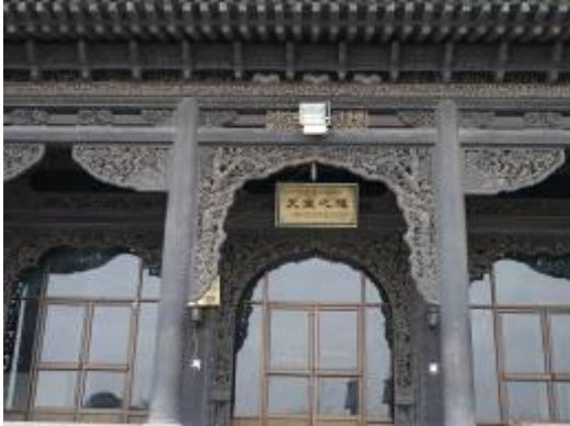
Figure9: decorated brace of Banqiao Mosque
