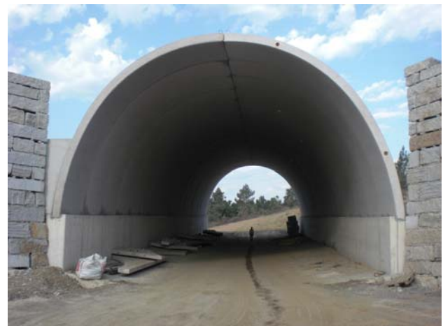
Figure 1. Underpass of Ourense – Celanova motorway (before backfilling process)
