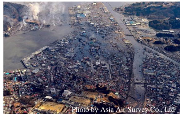
Figure 1. Kesen-numa city damaged by Tsunami
