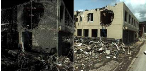
Figure 6. Two images of the holed building by tsunami – left: point cloud data, right: photography image
