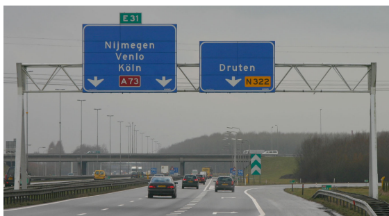
Figure 1. A typical traffic sign gantry on a Dutch highway with in the background a highway viaduct. The horizontal clearance is restricted by guard rails on both sides of the road. (Source: Rijkswaterstaat, 2006)
