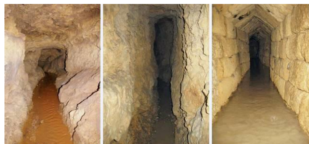
Figure 1. "Corso Gesuitico Alto". From the left, morphology of level 1, level 2 and level 3 sections of tunnels.
