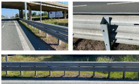
Figure 2. Identified insufficient levels of restraint during RSA on the D5 motorway (Prague – Nuremberg)
