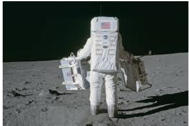
Figure 5. Buzz Aldrin carries the seismograph & array of Lunar Ranging Retroreflectors (LRRR).
