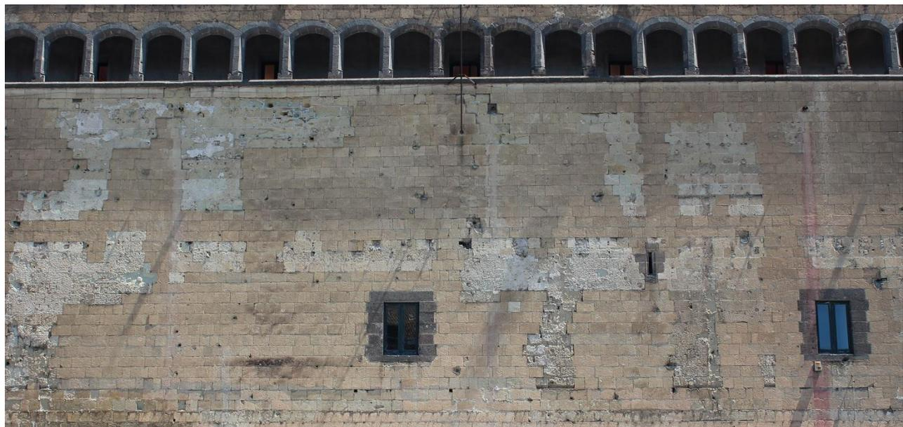
Figure 10. Castel Nuovo, Napoli. South Curtain: phenomenon of alveolization and retraction for erosion of the tuff surface. Unlike the uniformity connoting the image of the Castle, the walls show the heterogeneity of their surfaces which have been highlighted by specific representations.
