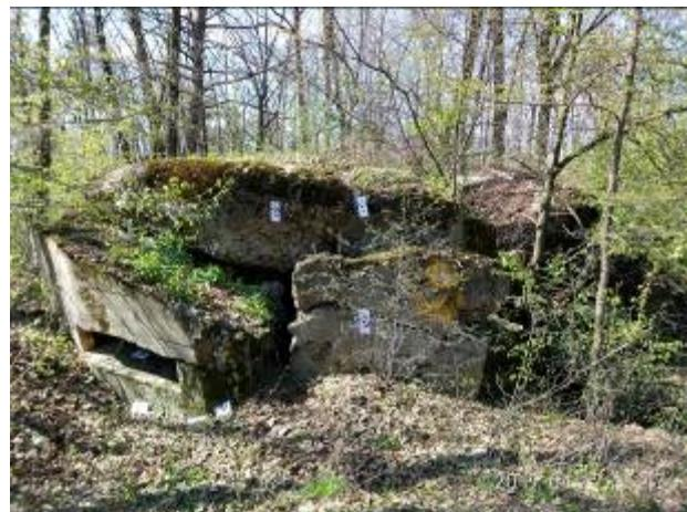
Figure 8. Image of pillbox № 451 with coded targets
