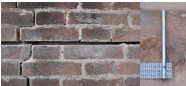
Figure 7: armed stitching along the mortar joints to close the cracks
