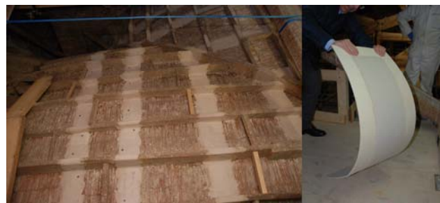
Figure 8: consolidation of the vault with bandages
