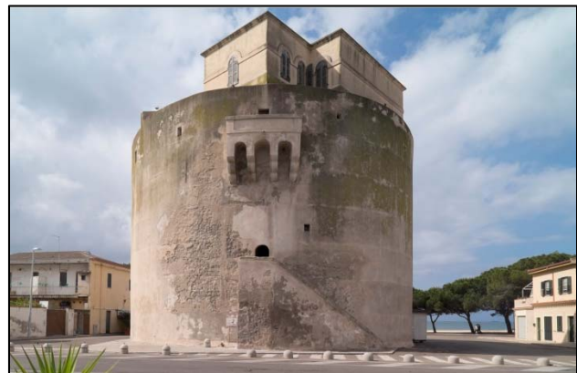
Figure 3. The Gran Torre of Oristano
