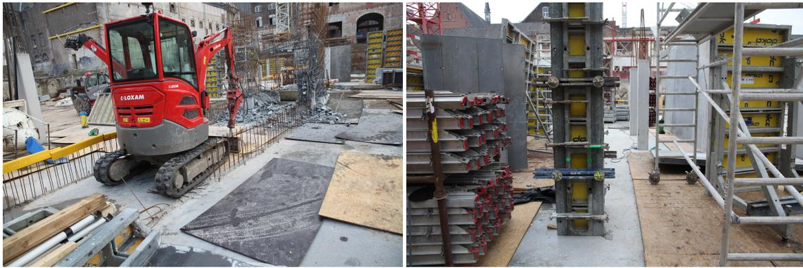
Figure 1: Auxiliary equipment and clutter on a construction site causing occlusions and registration errors
