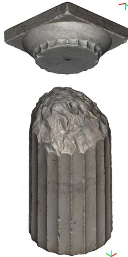
Figure 1. Doric capital and bottom column drum, which belong to the Nicias Monument. Point clouds produced with Agisoft PhotoScan®
