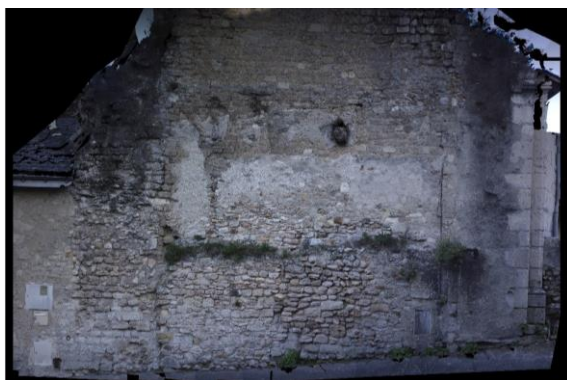
Figure 8. Orthoimage of the west wall of the north transept church
