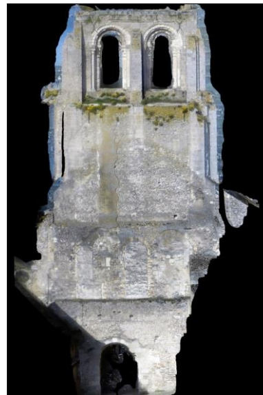
Figure 9. Orthoimage of the east face of St Paul tower
