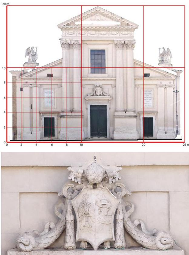
Figure 6. Final orthoimage of the whole façade with metric scale and sculptural detail above the main portal.
