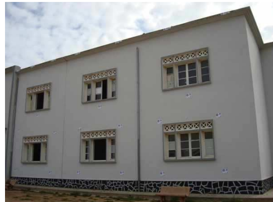
Figure 5. Targets distributed on the façade.
