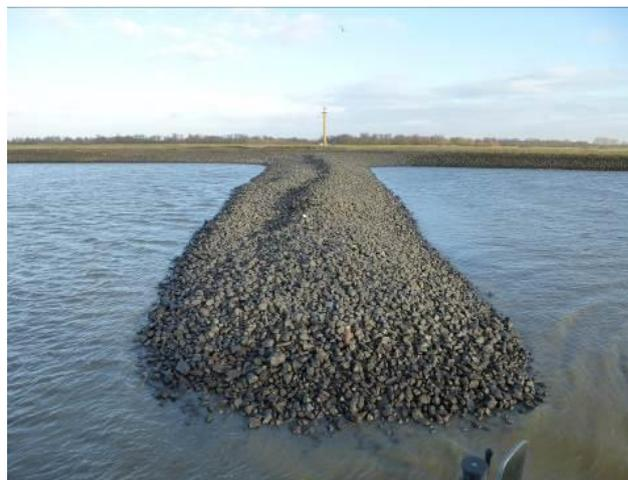
Figure 2. Damages despite optimized groyne design and construction
