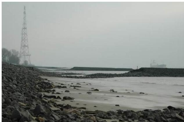
Figure 1. Breakthrough between groyne and revetment connection at Juelssand due to vessel-induced long-periodic wave loads
