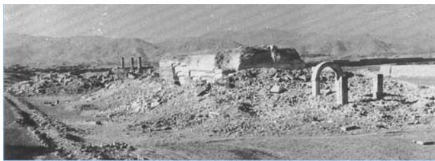
Figure 4. Exposed site of rammed earth station after the block collapse at 1940s
