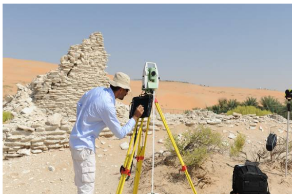
Figure 9. Monitoring survey of a major crack with total station at Om Hosn site in Liwa.
