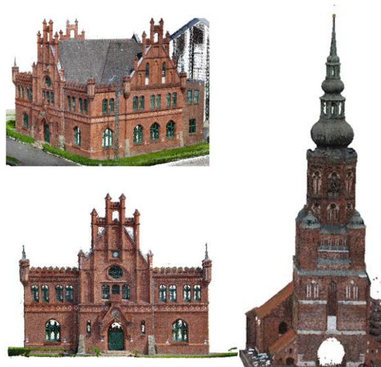
Figure 4. The generated point cloud of first dataset, whole of building (left and up) and the selected side for modelling (left and down), The generated point cloud of second dataset (right)
