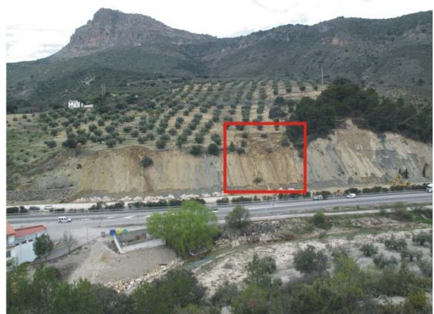
Figure 2. Panoramic photograph of studied landslide affecting road cut and upslope. The main scarp is inside the red square.
