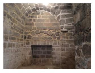
Figure 12. The geometry and stereotomy of the inner vaults and their intersections evidence a construction with a varied repertoire of solutions and techniques.
