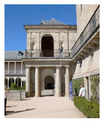
Figure 6. Differences of height between the external station points were directly measured with tape and plumb. Increases lately added were taken into account, as well as the difficulties introduced of the sloped wall of the Monastery's south façade.
